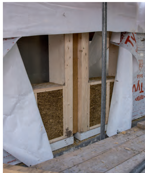
Prefab stropanelen achter folie.
